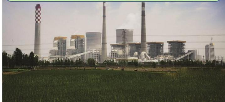
*A remarkable retrofit at Xuzhou Unit 3 boosted the 320-MW subcritical coal unit's efficiency to beyond 43.56%—higher than all existing Chinese supercritical units, and even many ultrasupercritical units. The groundbreaking demonstration is a POWER*
